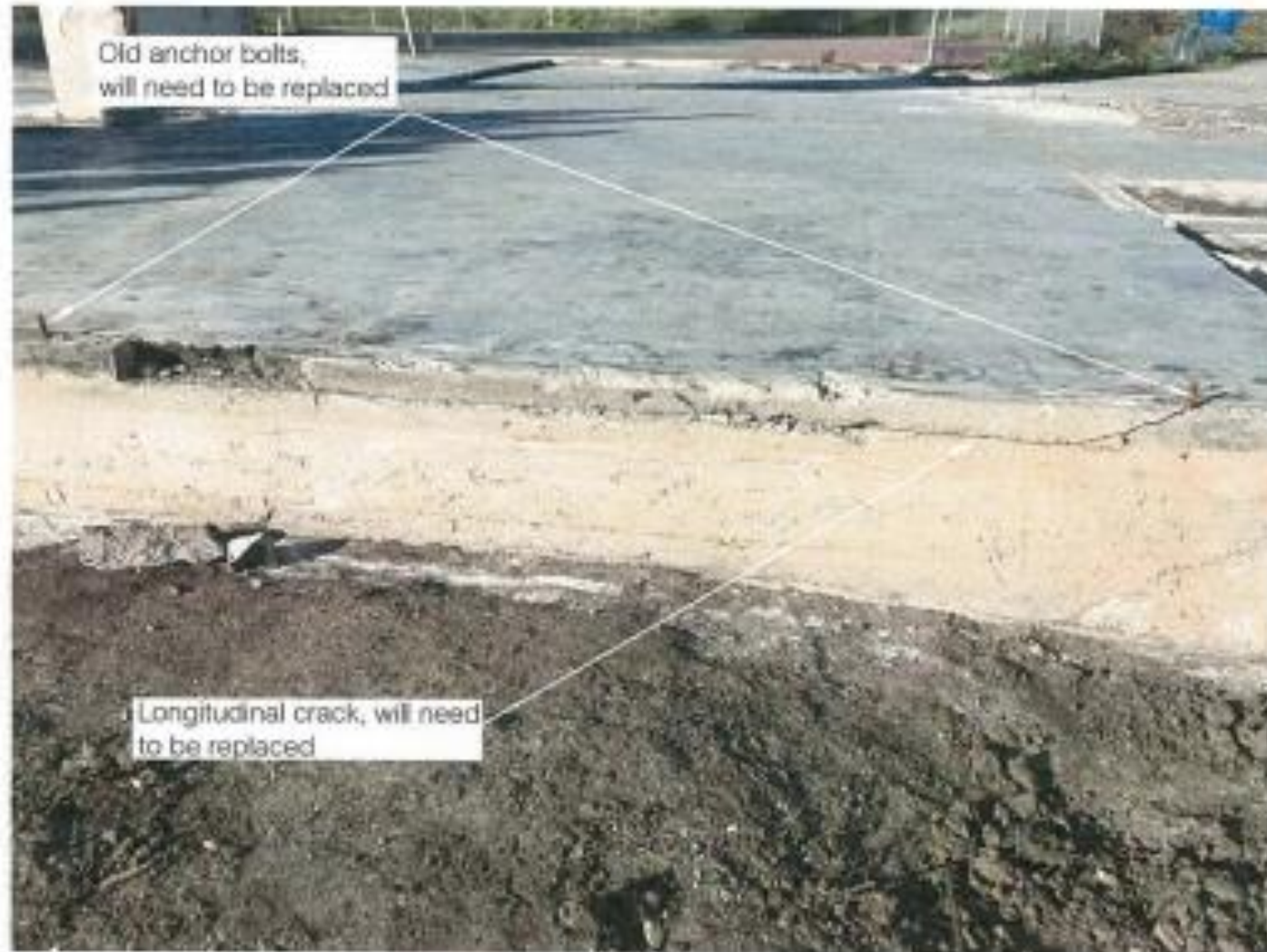
Site Photograph F
